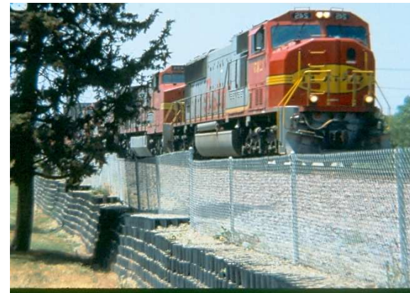
ROW Earth Retention
